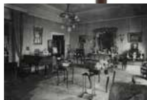
In situ in 94 Merrion Square, Dublin
